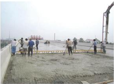
Bridge Construction Site
